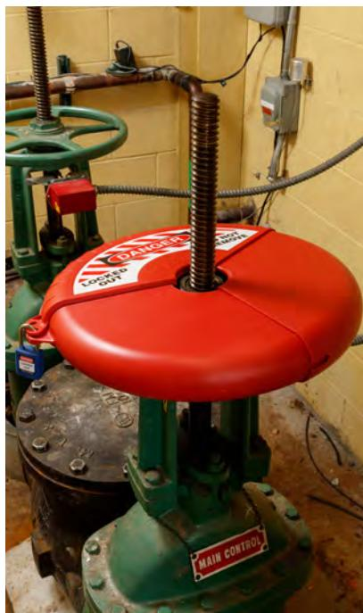
Brady's collapsible gate valve design provides secure lockout for a wider range of valves, with the use of fewer devices. These covers easily rotate around valve handles to the fully engaged position, while also folding into smaller sizes for easy storage on maintenance carts and in lockout kits.
