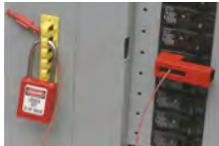
4. For group lockouts, run key through multiple loops in lock rail and apply locks. No hasps required! (Not recommended for use with multilock hasps)
