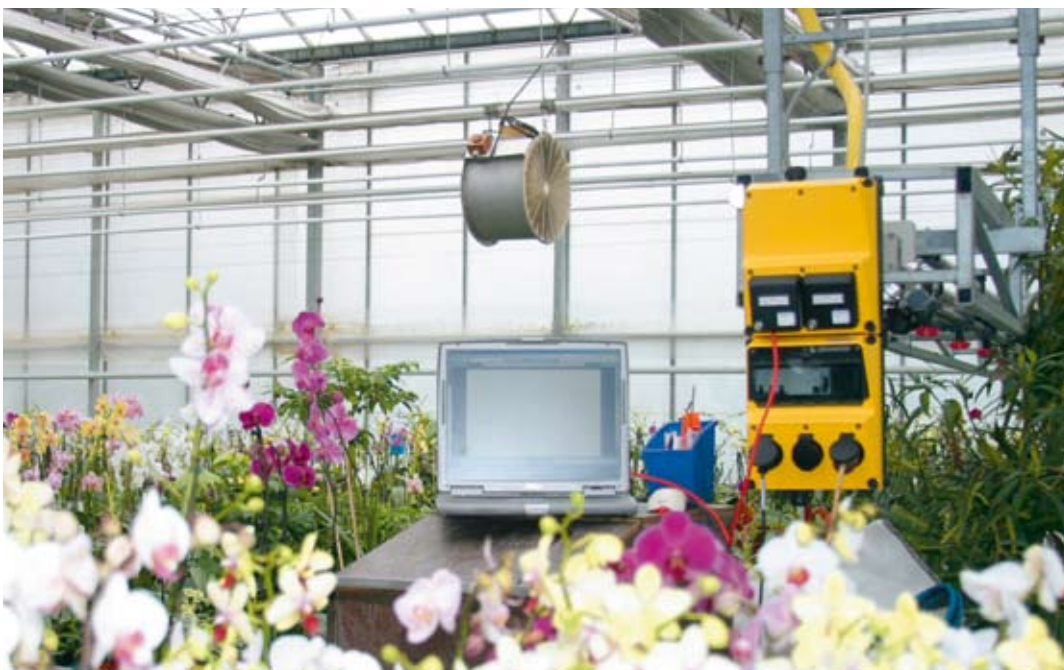
AMAXX network enclosure for safe installation in humid areas.
